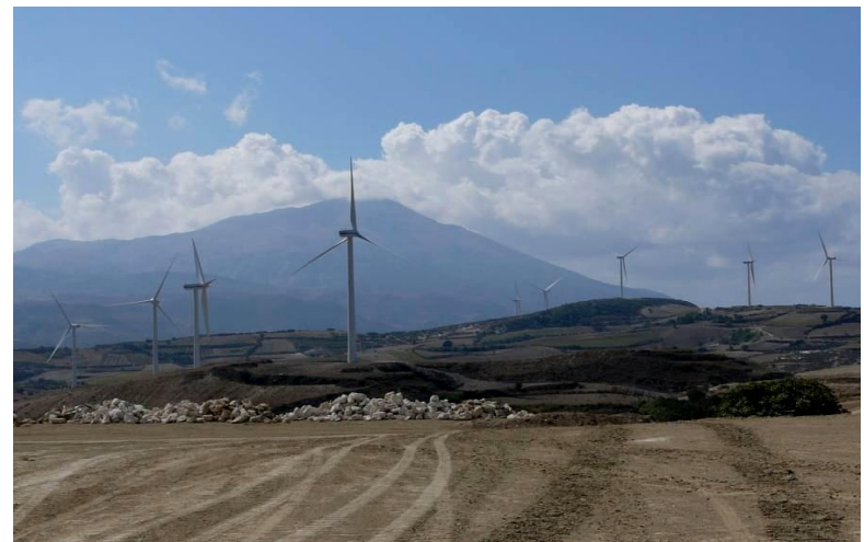
30 MW (15 x 2.000 kW) Windpark in Hatay Deniz A.Ş. (2007)
